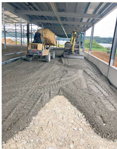
Groundworks for the Frutura farm by DMP.
