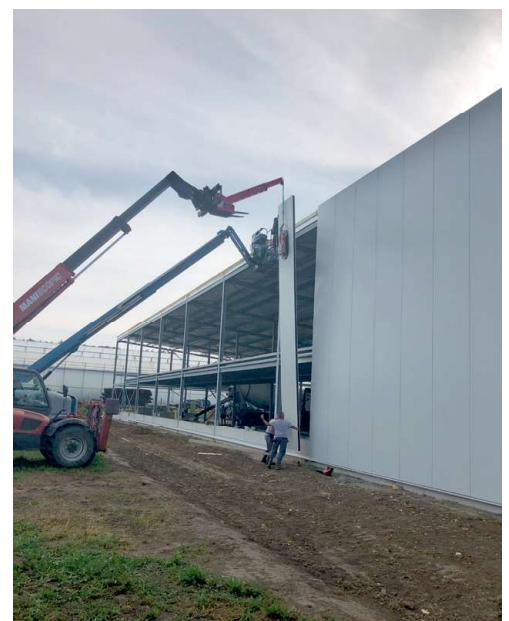
Building the farm: installation of cladding.
