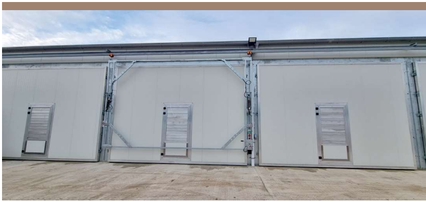
DMP filling door with door lifting system. The emergency doors have overpressure louvres.
