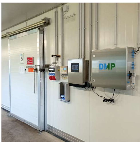
The Vec41 computer, especially designed by DMP for mushroom farms, and CO 2 multiplexer.
