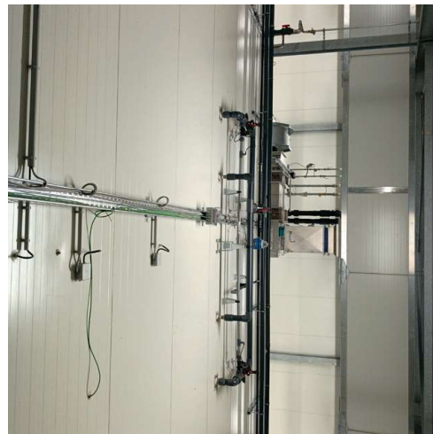
The farm has an in-bed watering system (left) and a tree watering system. Both watering systems are used to create the optimal, targeted watering for the mixed brown/white situation in the growing rooms.
